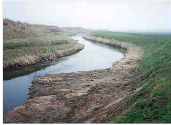
Figure 9 : Deflector on river Idle
