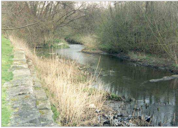
Figure 8 : Deflectors on river Wraysbury
